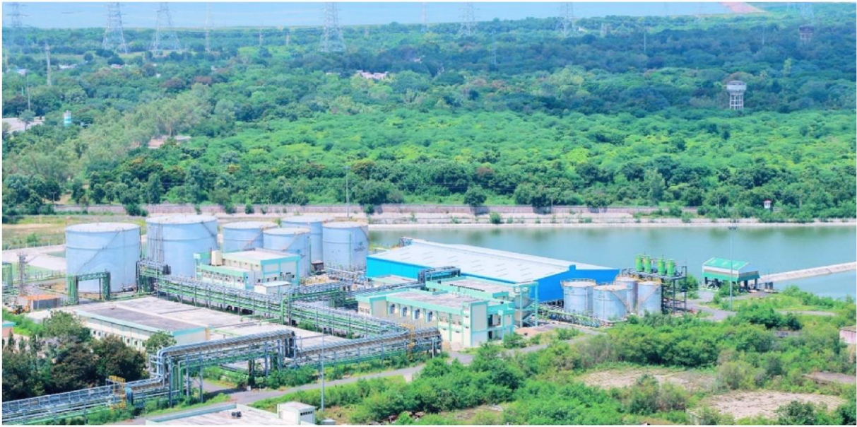
- RFCL Plant site aerial view, Ramagundam.
